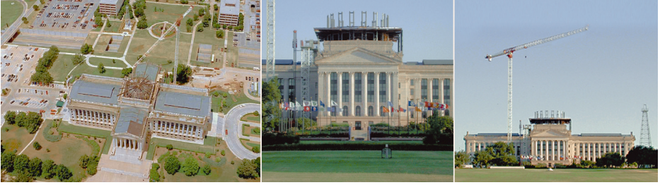
Early construction of the high dome involved the installation of the structural steel with the use of a tower crane 280 feet tall.
